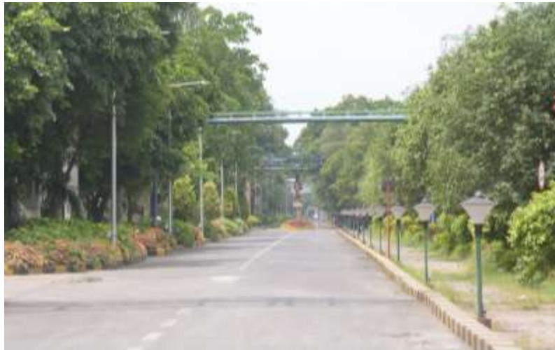
THERMAL POWER PLANT AREA
