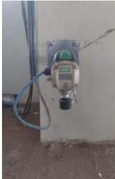
Fig. 2 Chlorine Sensors
