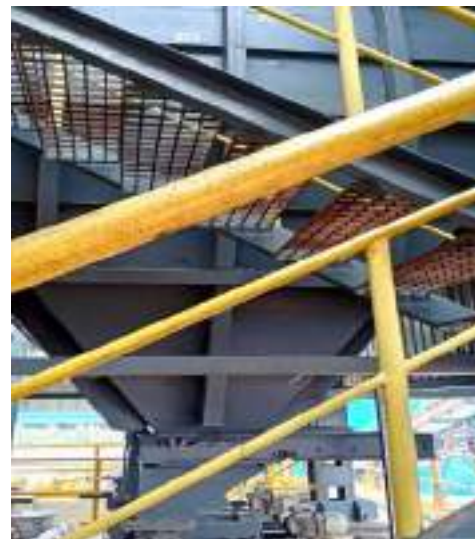
Fig 3. Bag filter installed at Coal transfer tower.
