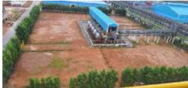
Fig. Greenbelt Chlorine bullets area.
