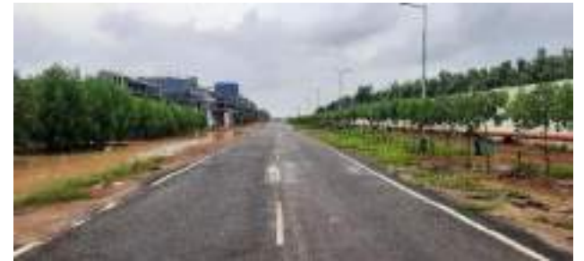
Fig. Greenbelt 15 TPH boiler area.
