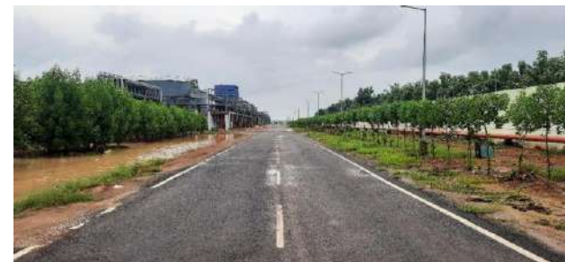
Fig. Greenbelt 15 TPH boiler area.
