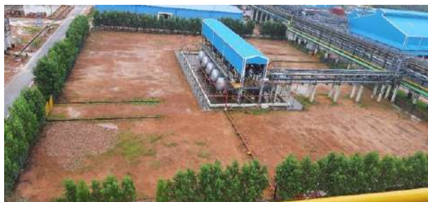
Fig. Greenbelt Chlorine bullets area.
