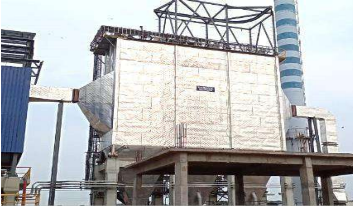
Fig 1. ESP connected to 15 TPH Steam boiler
