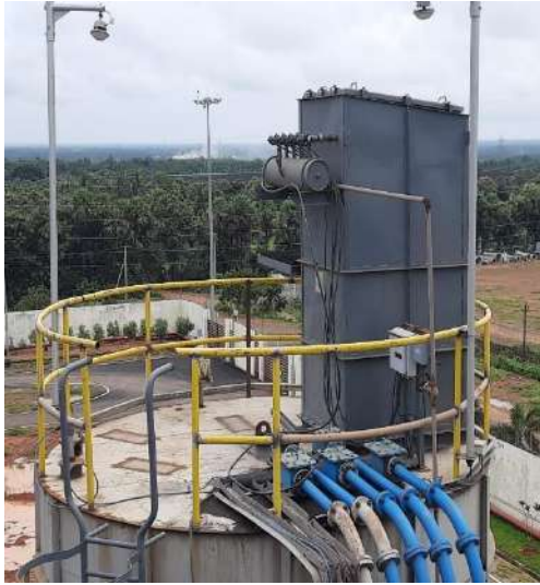
Fig 3. Bag filter installed at Fly Ash Silo
