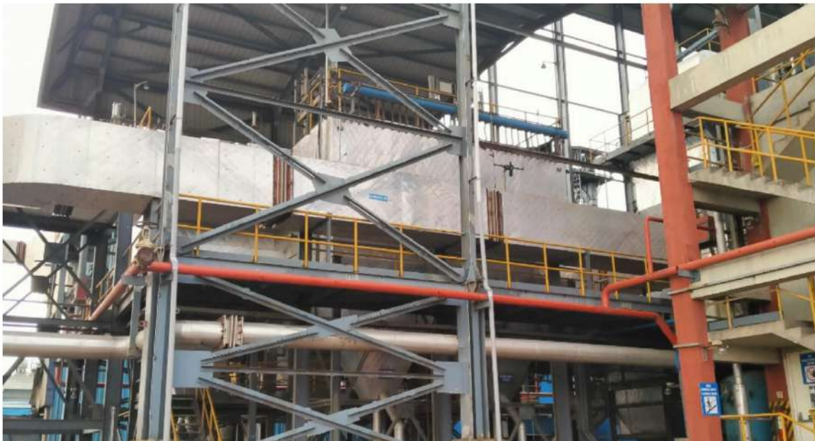
Fig 2. Bag Filters connected to 20 TPH Steam boiler
