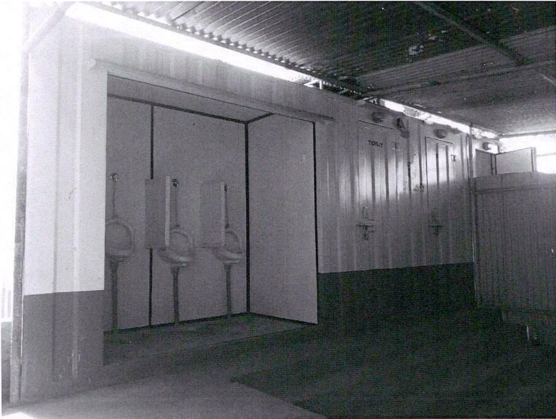
Mobile Toilet Facility Provided at Site
