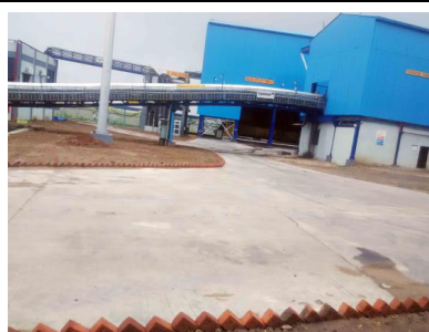
concreted Approach Road &amp; covered conveyor belt
