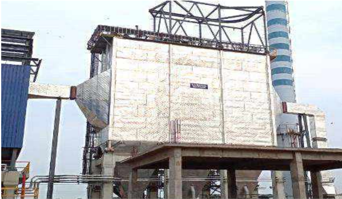
Fig 1. ESP connected to 15 TPH Steam boiler
