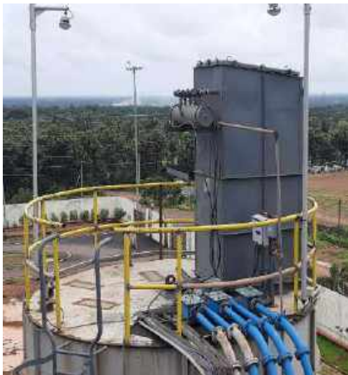
Fig 2. Bag filter installed at Fly Ash Silo
