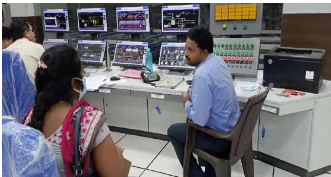
Fig2. DCS control room for carrying out remote operations for entire CAPS (Chlor Alkali products)
