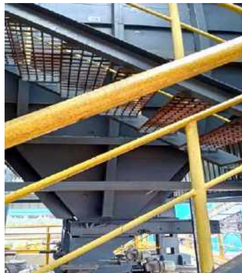
Fig 3. Bag filter installed at Coal transfer tower.
