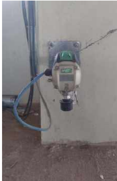
Fig. 2 Chlorine Sensors
