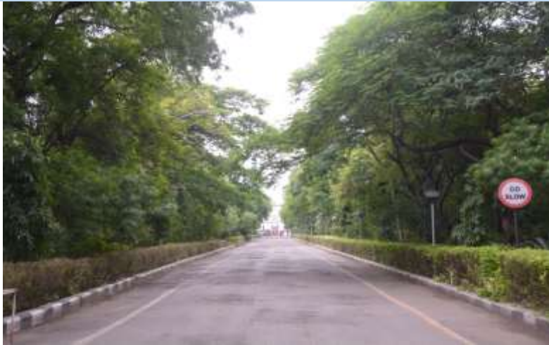
POWER HOUSE GATE
