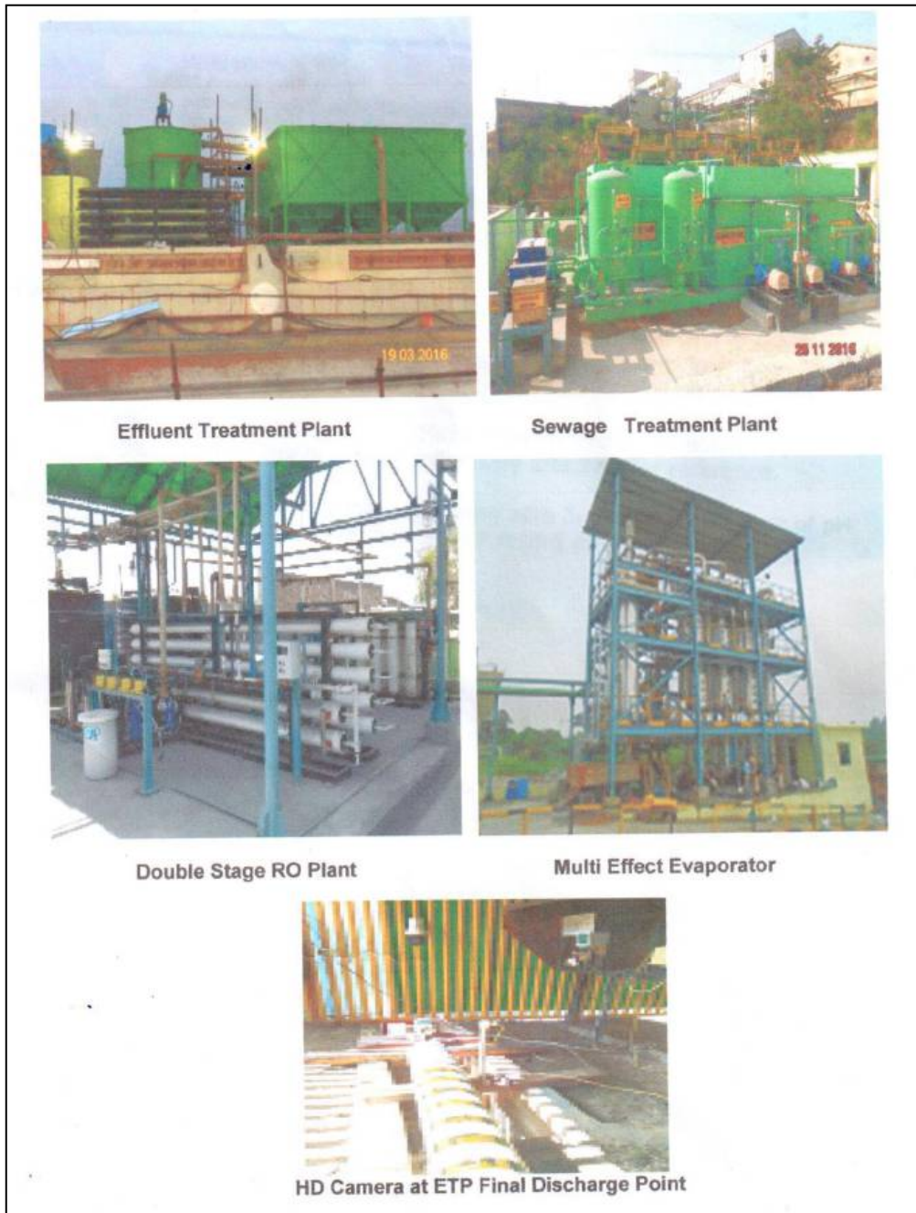
Figure 2.11: Photographs of ETP, STP, RO, MEE and HD Camera ETP final discharge point
