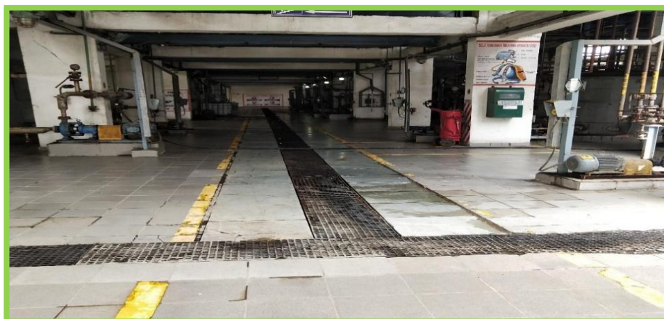
Figure no:24 Provision of Garland Drain
