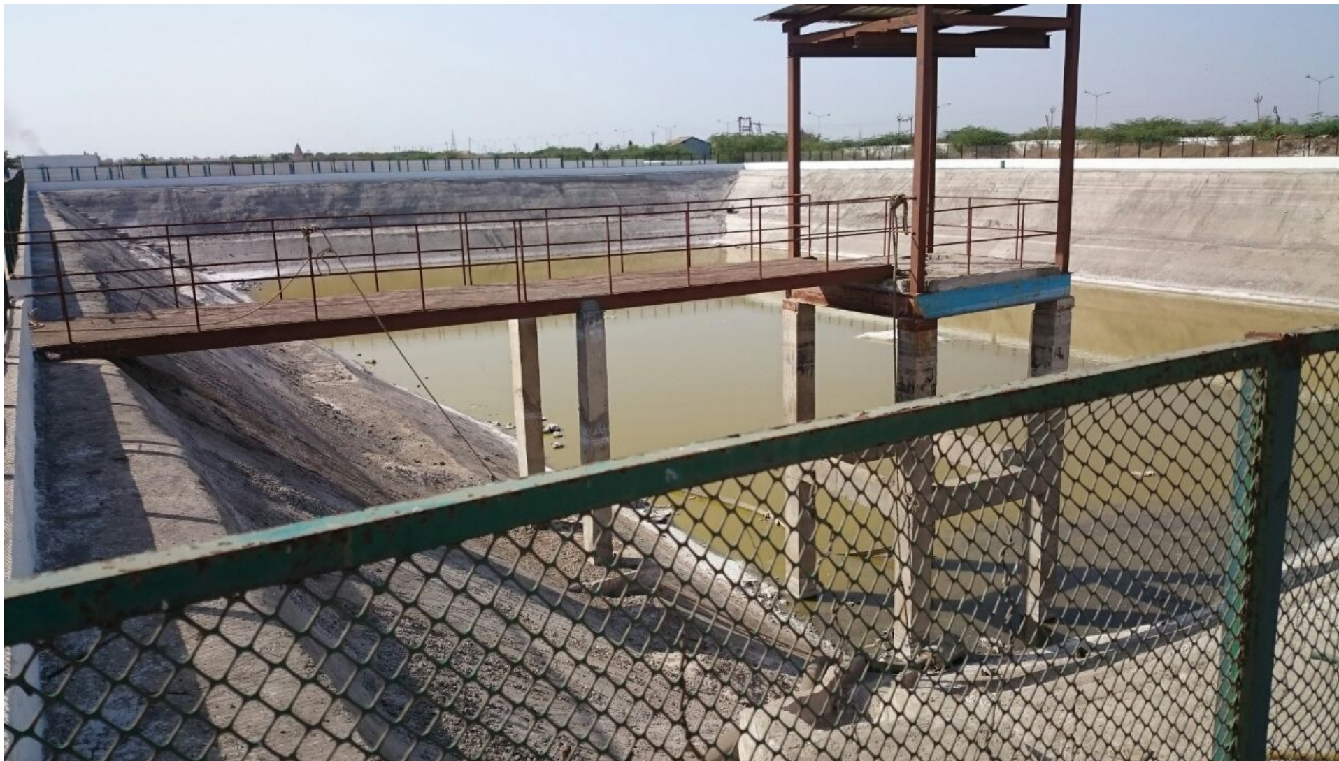
Figure – 01: - Guard pond for storage of Treated effluent
