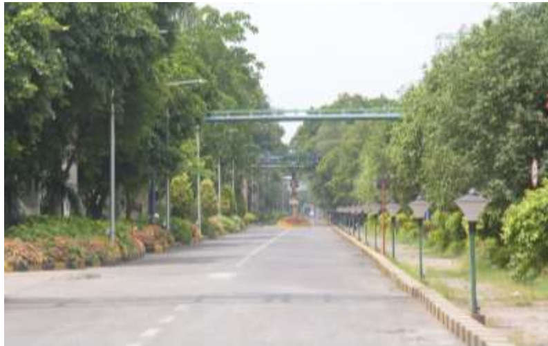
THERMAL POWER PLANT AREA
