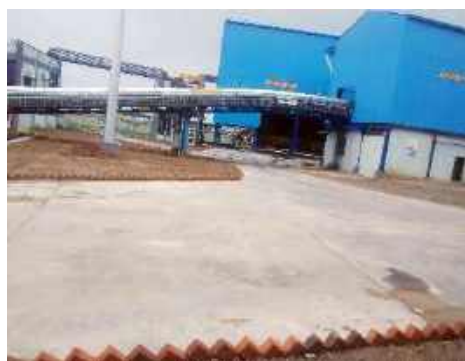
Concreted Approach Road & covered conveyor belt
