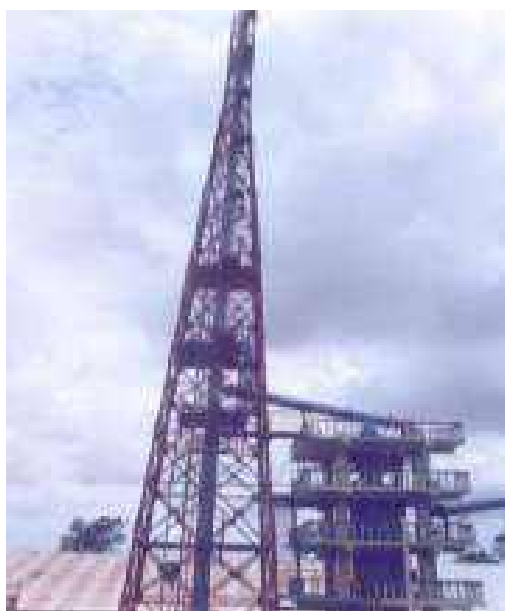
Sulphuric Acid Plant Stack with Alkali Scrubber & Demister to reduce SO 2 emissions and sulphuric acid mist respectively.
