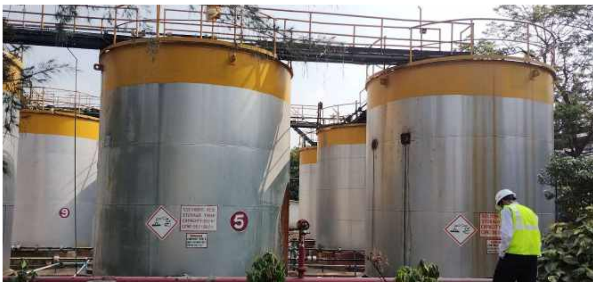
Sulphuric Acid storage tanks
