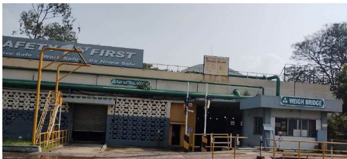
Raw Material Storage facility
