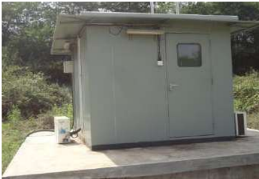
Figure 2 AAQM Station at Intake-well
