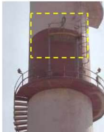
Power Plant Stack
