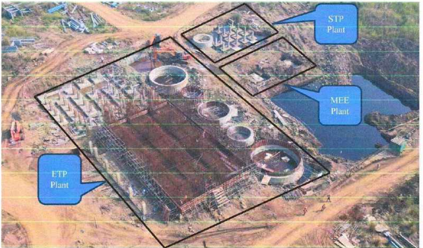
Construction site of ZLD Plant (ETP, RO, MEE) & STP Plant
