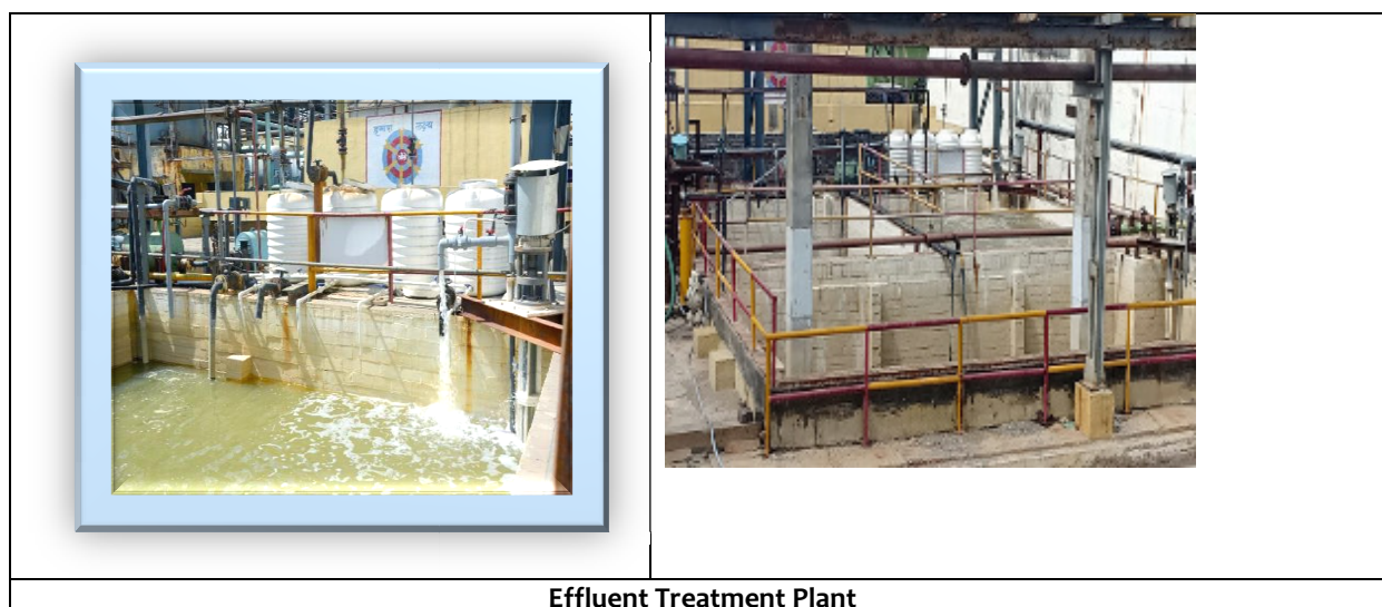
Effluent Treatment Plant
