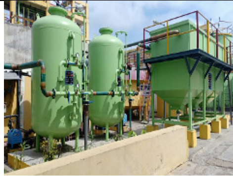
Lamella Clarifier with Sand & Carbon Filter
