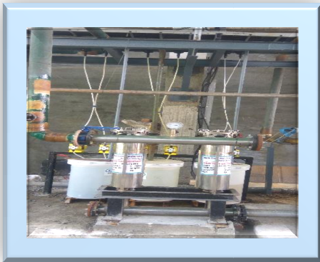
Chemical Dosing System
