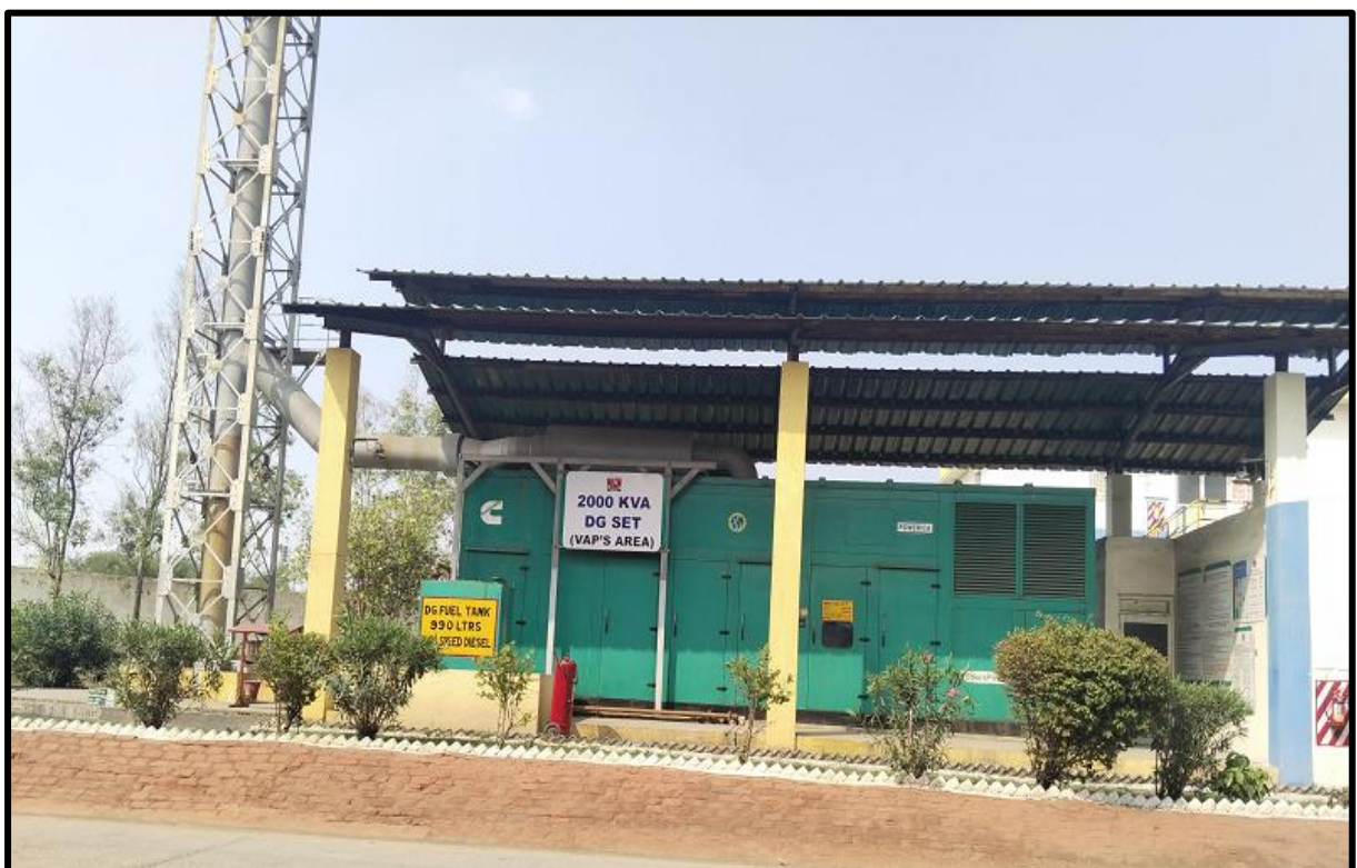
Acoustic Enclosure of DG set
