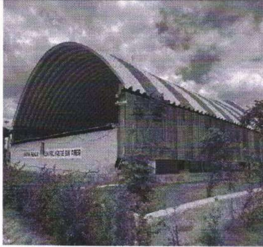
Photographs: Waste Storage Area
