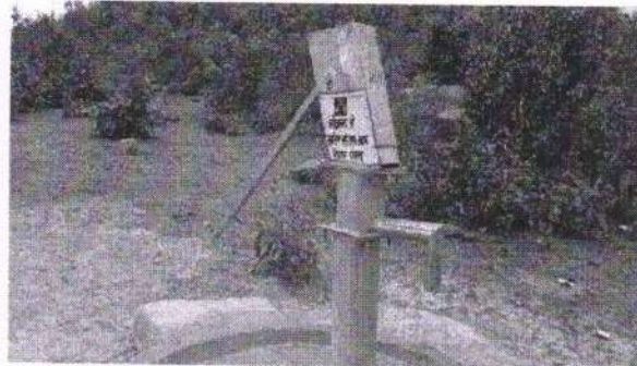
INSTALLATION OF HANDPUMPS
