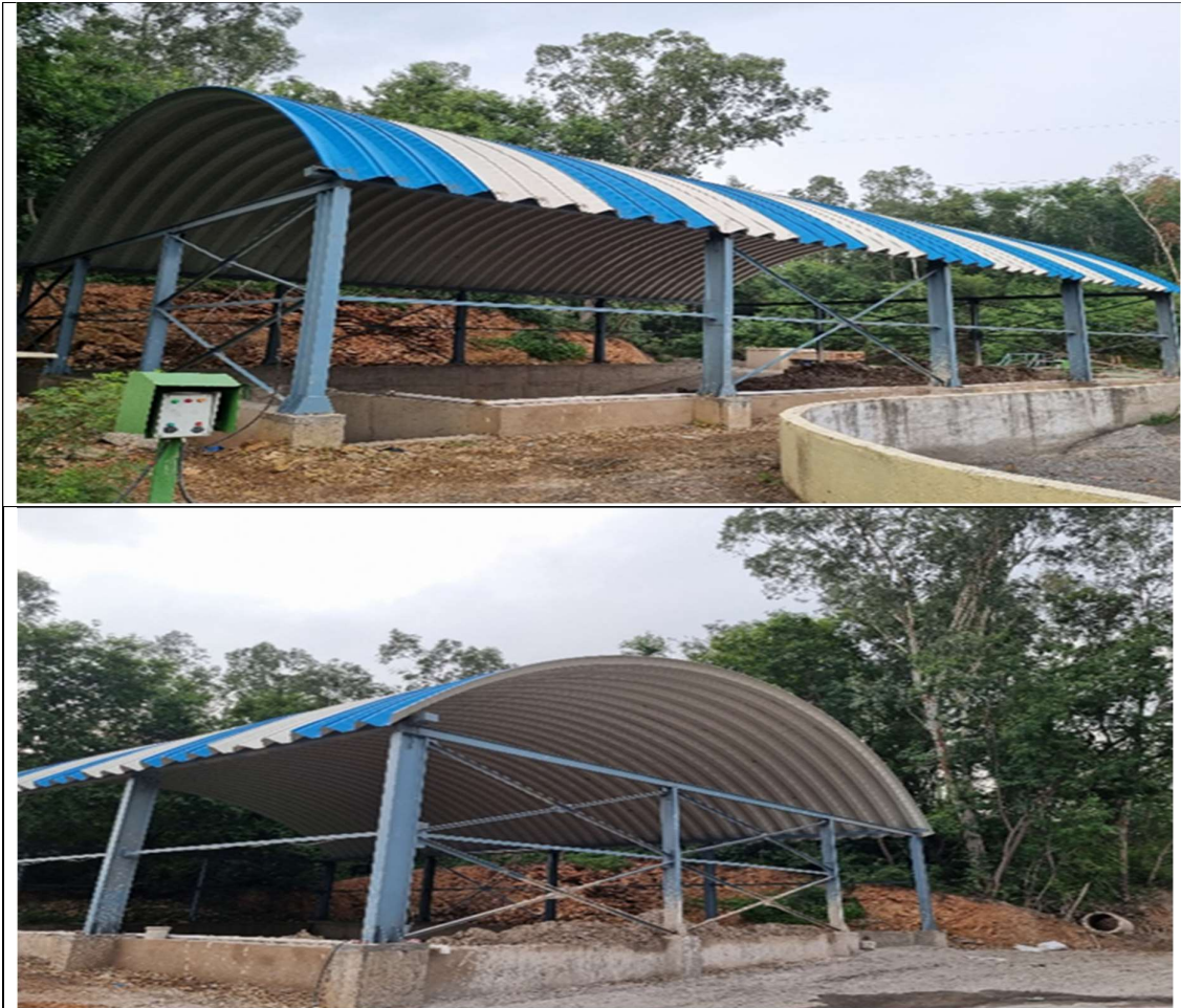
Picture: Hazardous waste storage area at GRCD
