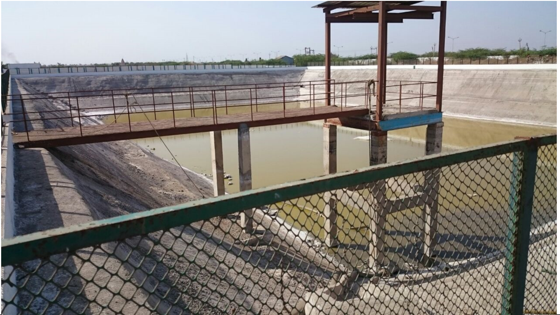
Figure – 01: - Guard pond for storage of Treated effluent
